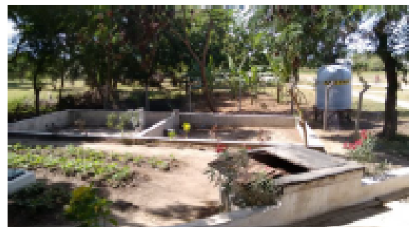
Figure 3: Onsite DEWATS Facility
