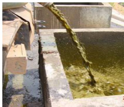
Photo 3: Fresh FS collected from unsewered public toilets unloaded at Buobai FS treatment plant, Ghana. (Source: Eawag/Sandec, 2003)
