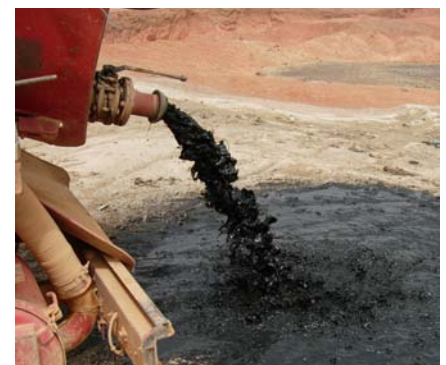
Photo 4: Discharge of untreated septage. (Source: Eawag/Sandec)
