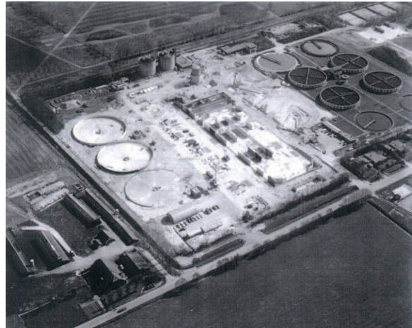
Figure 1.8 – Overview of a WWTP (under construction)
