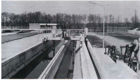
Figure 2.7 - Rectangular horizontal flow grit chamber
