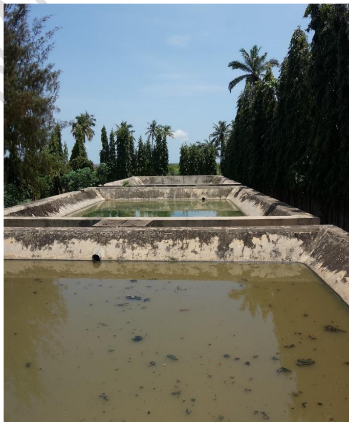
Photo: PATH Figure 15. DCAM Bethesda's graywater treatment pilot site.
