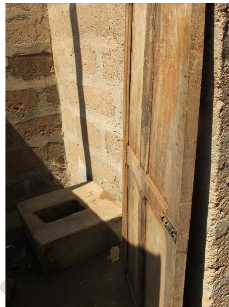
Photo: PATH Figure 5. Suggested improvements included additions and repairs to existing facilities, such as this latrine that is missing a roof and has a broken door that is sitting in the stall.
