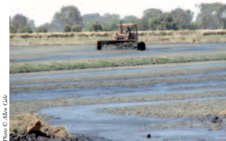
Figure 2. Mechanically assisted drying in bays at Shepparton WMF
