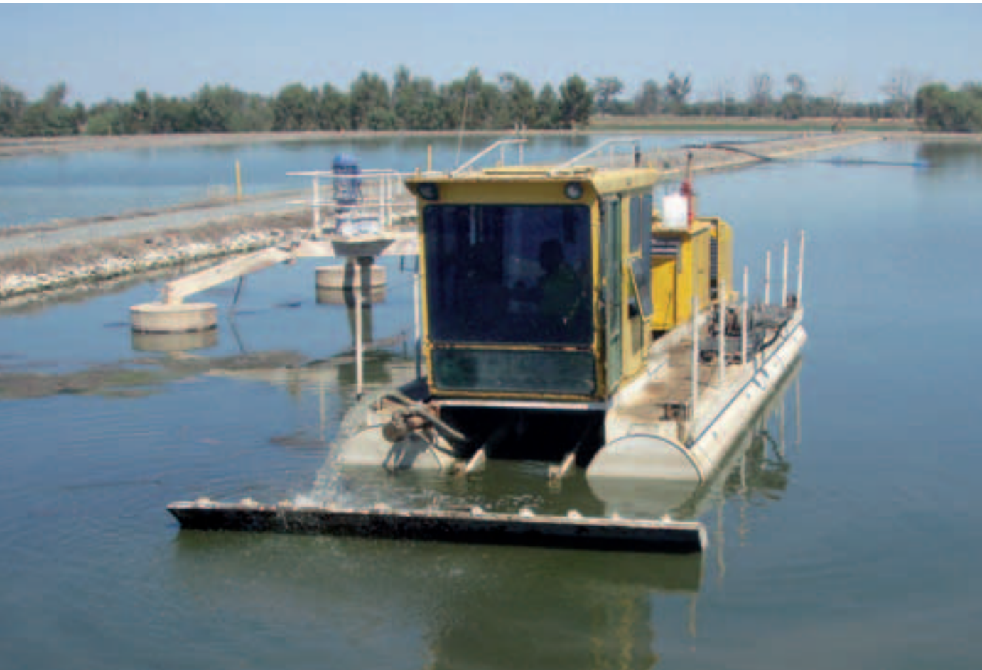
Dredge for Lagoon Desludging, South East Australia. Photo © Allen J Gale
