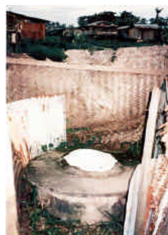
Photo 9 Pour-flush toilet with soakage pit in Vientiane, Laos (Photo J. Parkinson, GHK)
