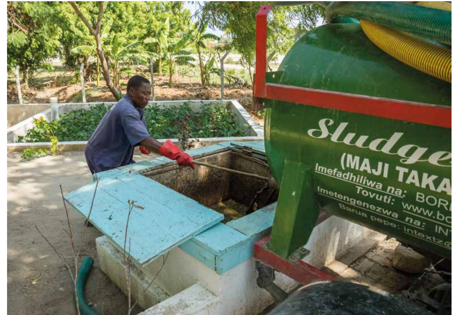
Kigamboni treatment plant →
