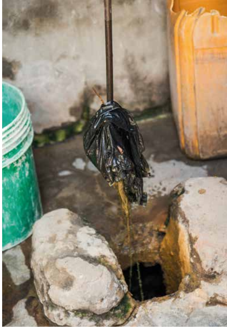
Removing plastic waste before pumping
