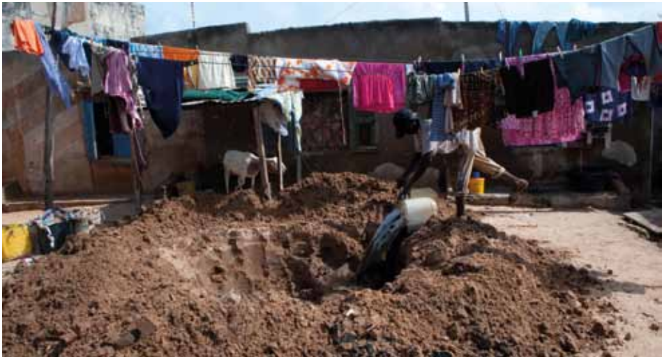
Figure 14.9 Faecal sludge manual emptying and burying within the courtyard (photo: Linda Strande).
