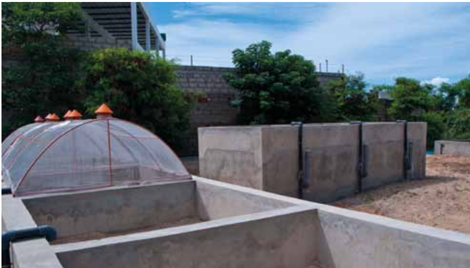
Figure 7.6 Pilot scale research facility at Cambérène treatment plant, Dakar, Senegal. Evaluating rates of dewatering with passive and active ventilation with greenhouses (photo: Linda Strande).
