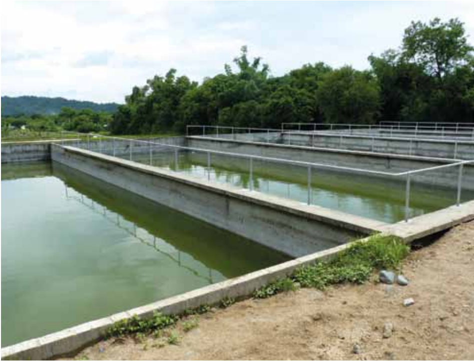
Figure 11.8 Starting up period of faecal sludge lagoon system, San Fernando City, Philippines. In this case, lagoon basins were seeded with activated sludge from a nearby wastewater treatment plant (photo: David M. Robbins).
