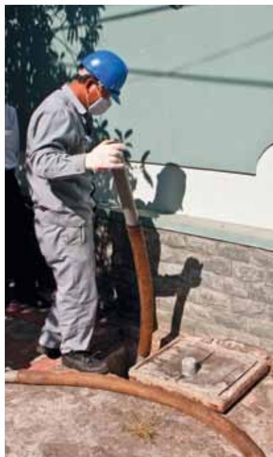
Figure 4.3 Example of a septic tank access port designed for ready access, Vung Tau Province, Vietnam (photo: Linda Strande).
