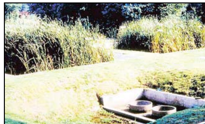
Photo 1: Cattail-planted constructed wetlands
