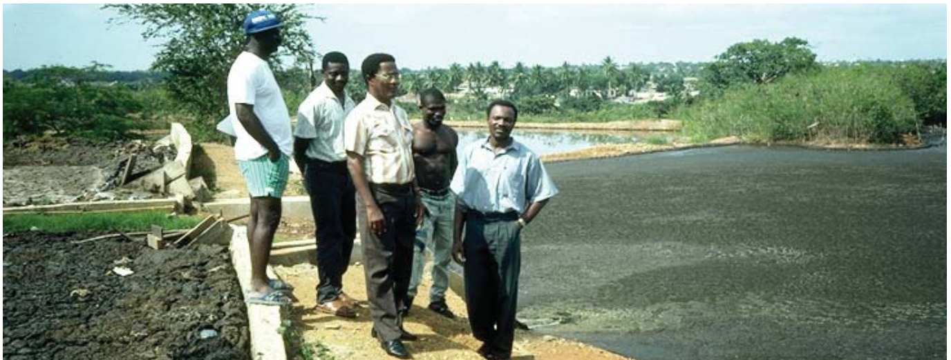
Photo 5: Ghanaian sanitation experts and treatment plant operator at an FS treatment plant in Ghana (left: FS settling-thickening tank; right: stabilization pond for settling tank supernatant)
