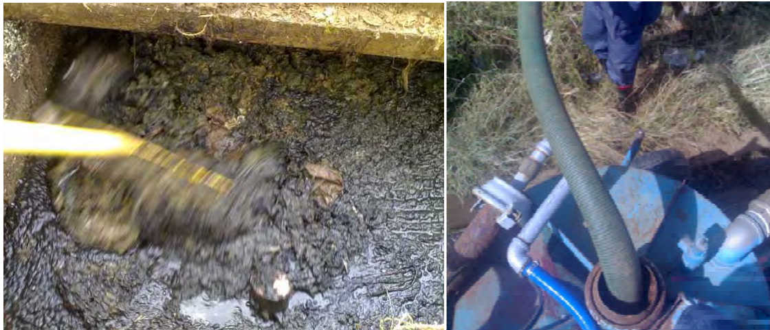
Figure 5.11 Rubbish being removed from a pit with a rake (left). Using the Vacutug hose to mix water with sludge inside the tank (right).
