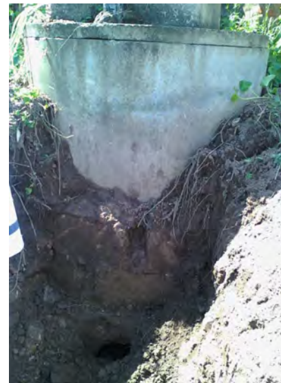
Figure 1.1 Some pits are difficult for workers or equipment to access
