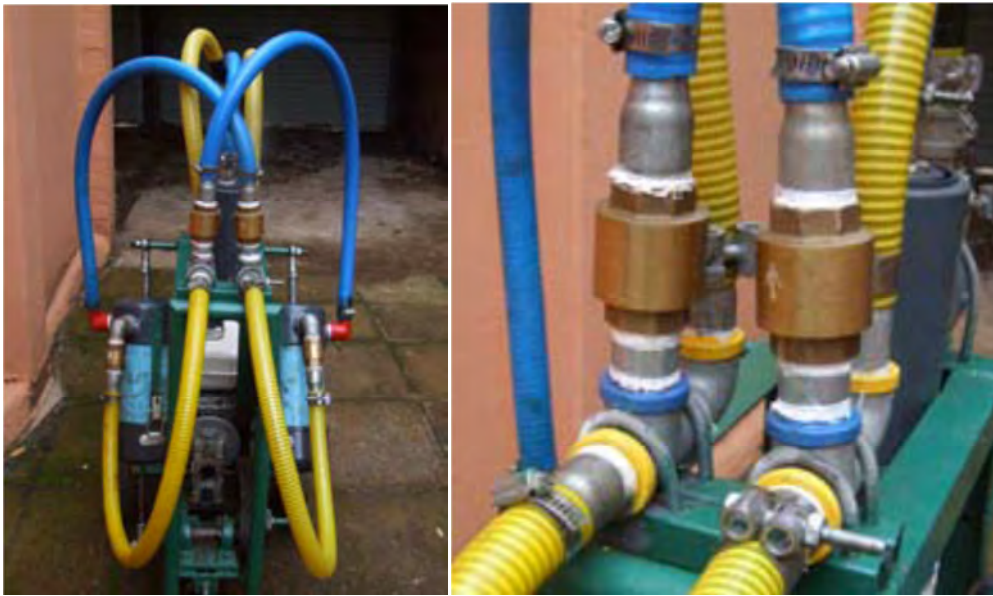
Figure 6.4 Configuration of pipes changed so that lower pipes are yellow and upper pipes are blue.
