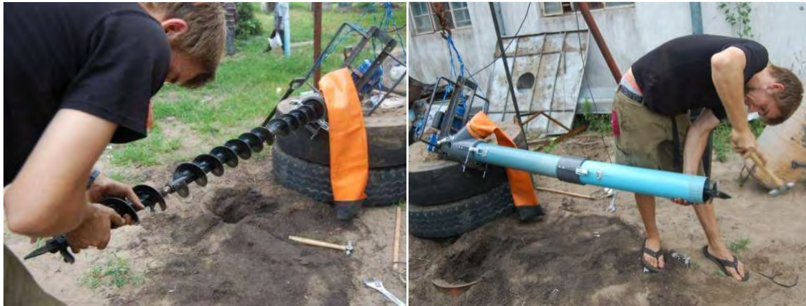
Figure 4.8 Adding an extension to the auger
