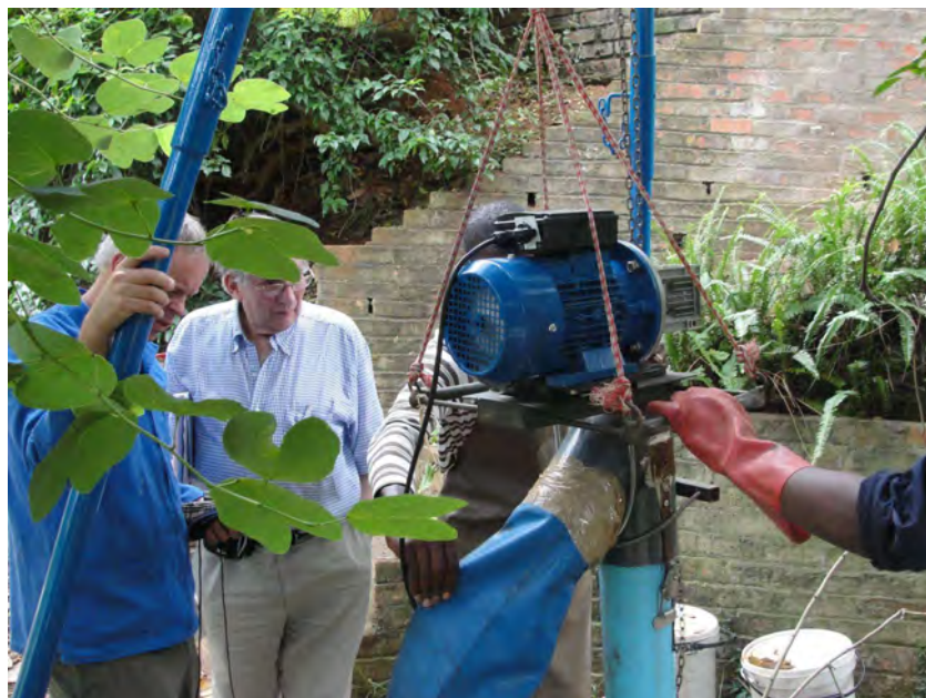
Figure 4.10 Pit screw auger during testing
