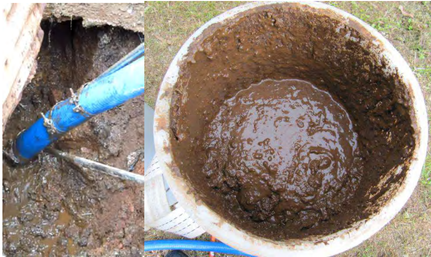
Figure 7.11 Emptying a pit with the eVac
