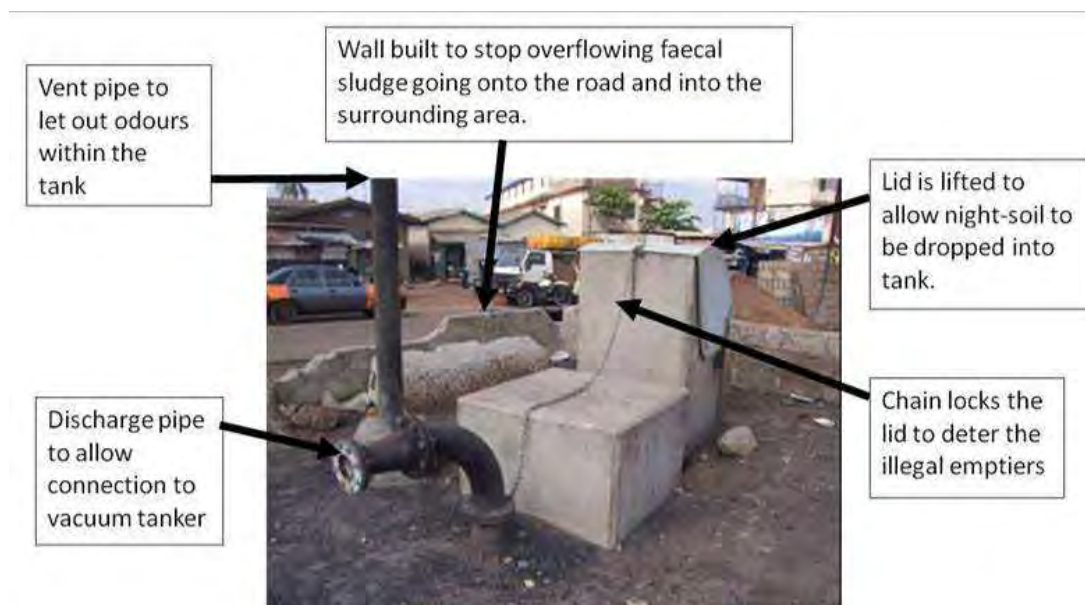
Figure 5.7 Transfer station in Ghana, (UN-HABITAT)
