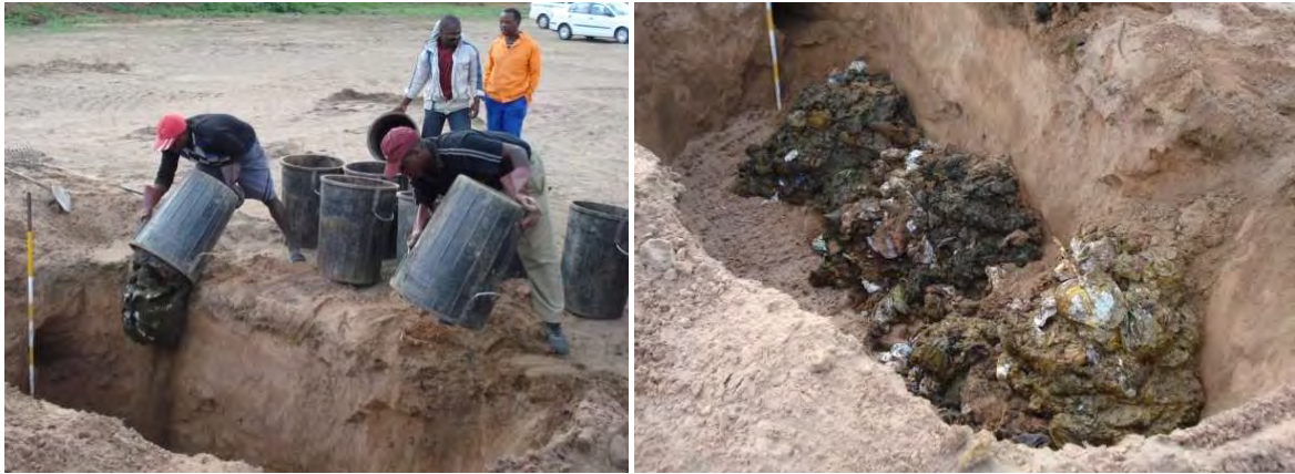
Figure 6.11 Pit sludge with high rubbish content buried in trenches
