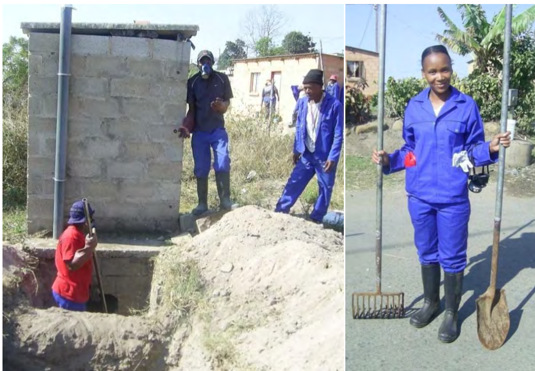
Figure 4.7 eThekweni pit emptiers at work
