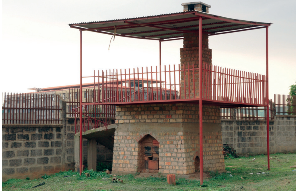
Figure 18.6 FaME (Faecal Management Enterprises) project pilot scale kiln for co-combustion of faecal sludge in brick production in Kampala, Uganda (photo: Pitman Ian Tushemeziwe).
