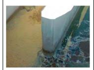
Figure 5: Fat, blood and feathers collected in one of the corners of chlorine contact tank
