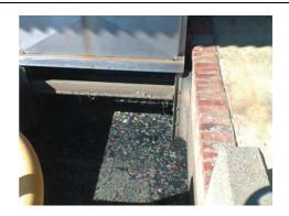
Figure 2: Bloody wastewater turning septic in one of the inlet screens due to blockage caused by "thick" clots of blood in the wastewater
