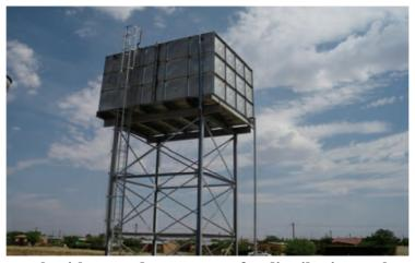
Figure 7: Storage tank with treated wastewater for distribution to the connected houses
