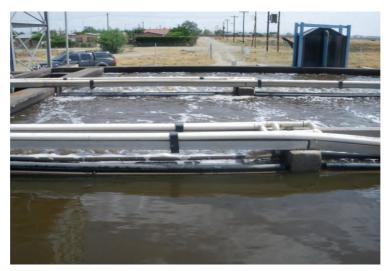
Figure 6: Tokologo – Close circuit wastewater treatment tank divide into three compartments of equal volume
