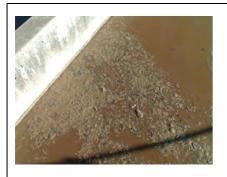
Figure 3: Feathers collected in one of the corners of the activated sludge reactors in Hartbeesfontein
