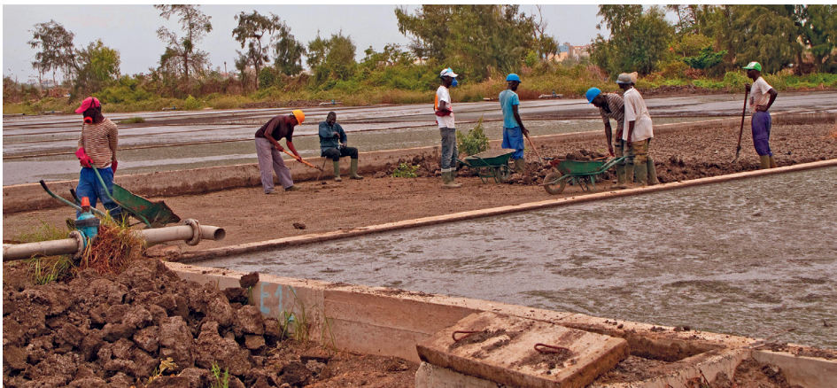
Figure 12.2 Harvesting of sludge from drying bed for use in agriculture, Dakar, Senegal (photo: Linda Strande).
