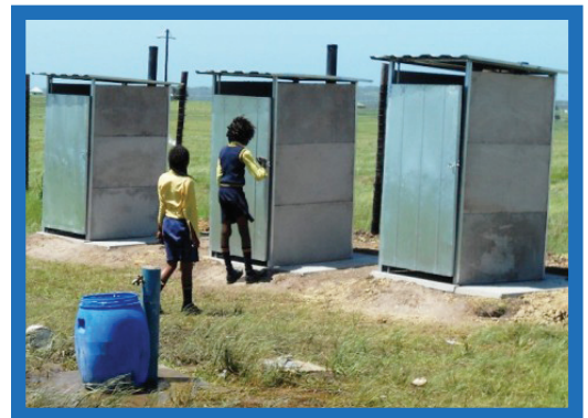
Brand-new toilets installed by the franchisees at two schools.
