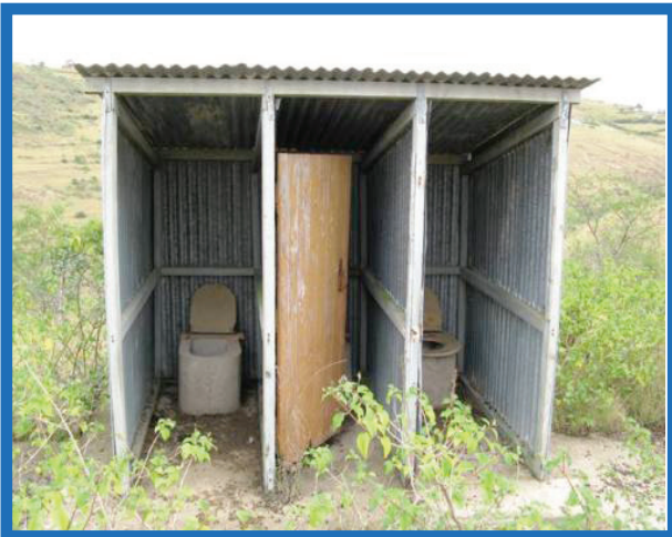
Left: Learners' cubicles unusable, with no door, and overgrown. Right: No roof to toilet block
