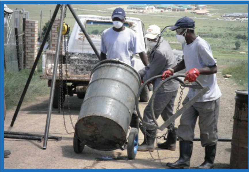
Moving the 200 L drum filled with material taken out of the household pits in Dutywa (ADM), to the disposal site.
