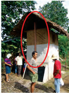
VENT PIPE TOO SHORT
