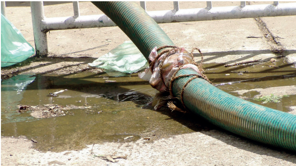
Figure 4.4 Hoses and fittings require frequent attention and repairs to keep them functioning properly. This picture illustrates inadequate maintenance, resulting in leaking of FS from the emptying hose (photo: David M. Robbins).
