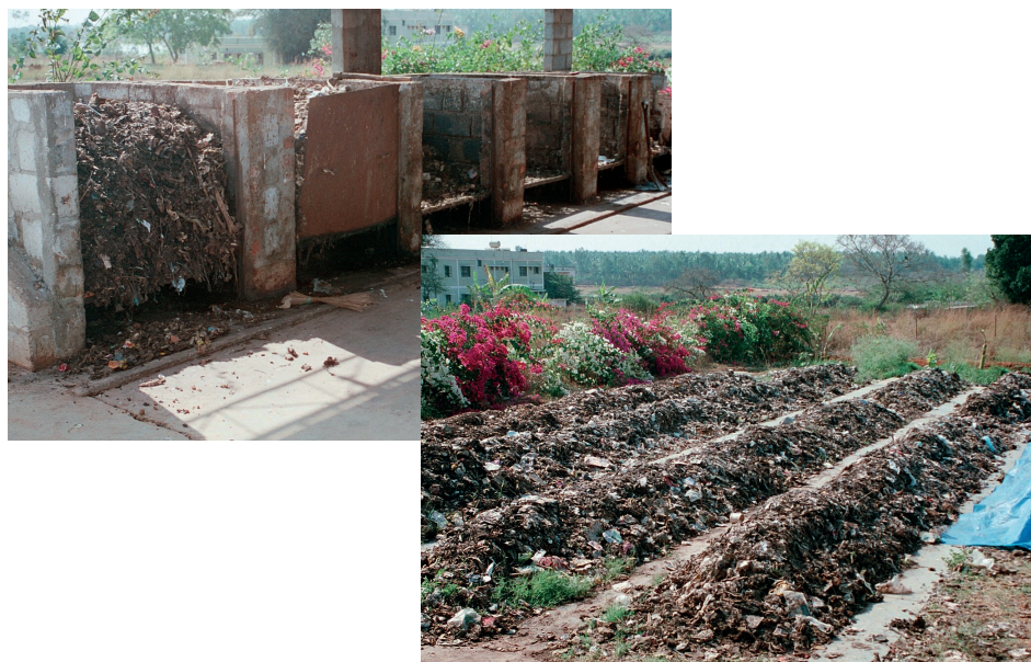
Figure 3.11 Pilot scale co-composting facility with faecal sludge and municipal waste in Bangalore, India (photo: Chris Zurbrügg).
