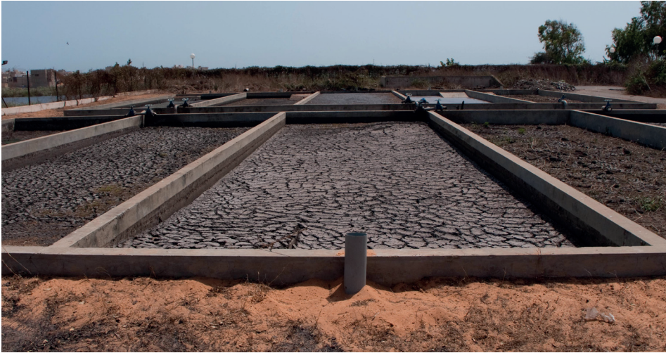
Figure 3.4 Drying beds at Niayes faecal sludge treatment plant, Dakar, Senegal (photo: Linda Strande).
