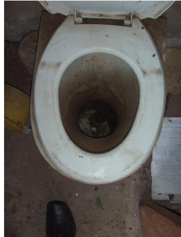
A full pit as seen from toilet
