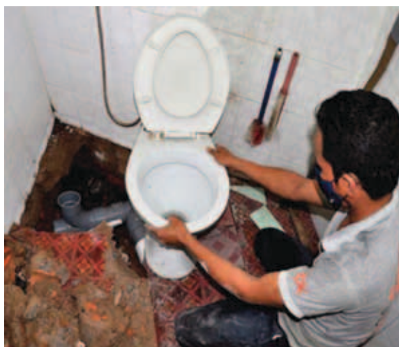
Figure 3.2 Connection of Household Sanitation Facilities to SSS
