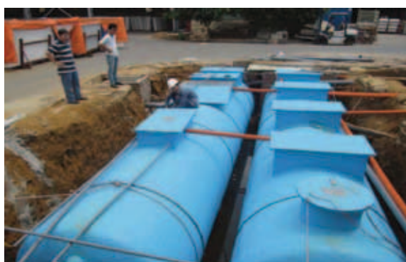
Figure 3.1 Decentralized, Pre-fabricated WWTP for the Office Building
