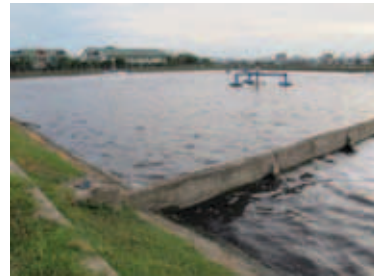
Diluted incoming flow from CSS makes installation and continuous operation of surface aerators unnecessary (Binh Hung Hoa WWTP, HCMC)
