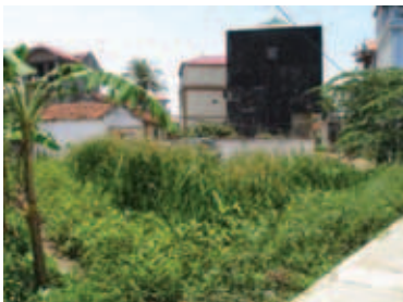
Baffled septic tank and constructed wetland systems in Lai Xa Village, Hanoi sub-urb
