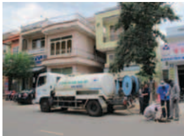
Sewer cleaning in Buon Ma Thuot city
