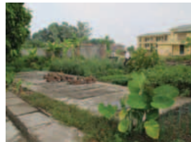
Decentralized wastewater treatment plant in Kieu Ky Village, Hanoi sub-urb
