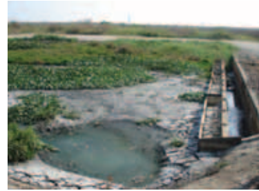
Settling pond for septage treatment in Trang Cat, Hai Phong
