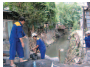
Manual cleaning of combined sewerage in Hanoi city
