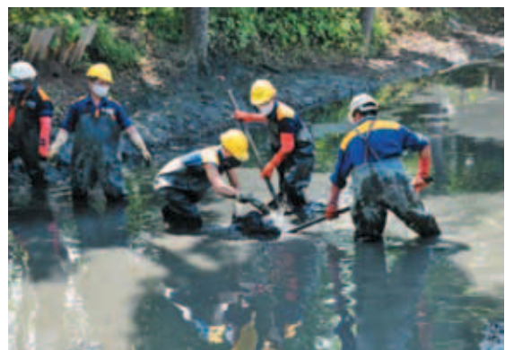
Figure 1.10 Cleaning of Urban Drainage Canal
