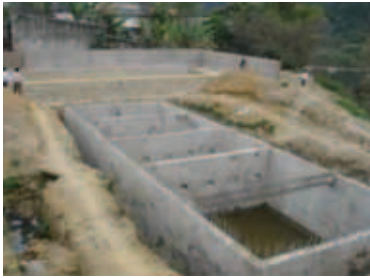
Baffled septic tank and constructed wetland systems in Cho Moi town, Bac Kan province
