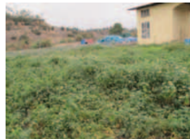
Septage treatment station with lime conditioning and drying beds (not in operation) in Ha Khau WWTP, Ha Long
