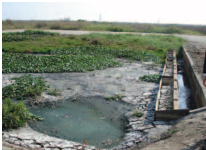
Figure C10: Settling Pond for FS Treatment in Trang Cat
