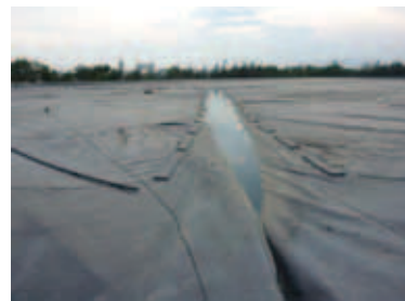
Due to rapid urbanization, this anaerobic pond has been covered. However, in order to meet effluent standard, the pond effluent will be soon pumped to the new WWTP for further treatment
