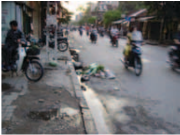
Open discharge of rainwater, grey water and septic tank effluent to street is a common picture in most cities
