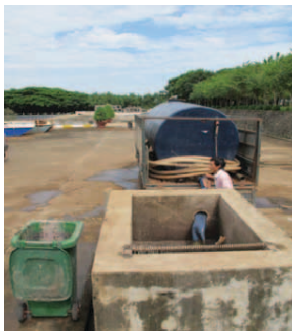
Figure C13: Septage Pumper Truck Off-loading to Septage Receiving Station at WWTP (Buon Ma Thuot City)
