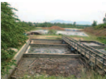
Septage thickening at Khanh Son waste treatment landfill, Da Nang
