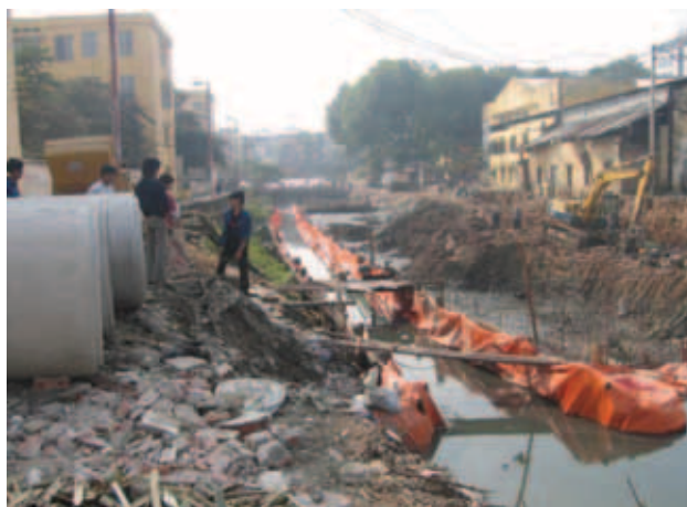
Figure 1.2 Construction of drainage canal in Hanoi City
