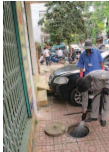
Household connection manhole is being cleaned in Buon Ma Thuot
