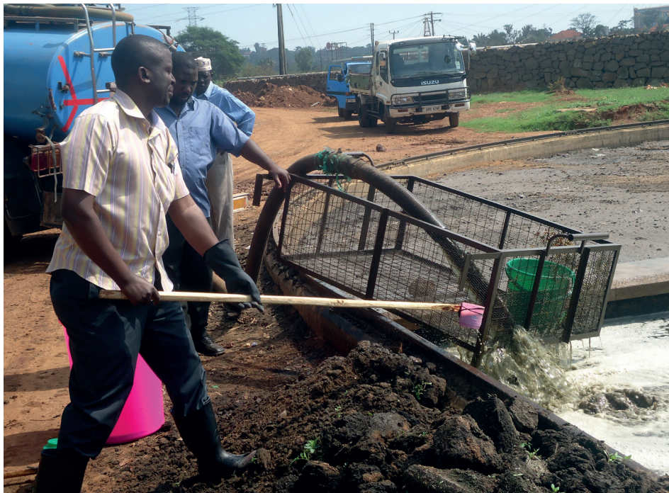
Figure 2.5 Municipal solid waste removed from faecal sludge with bar screens at treatment plant influent during a sampling event in Kampala, Uganda (photo: Daniel Ddiba).
