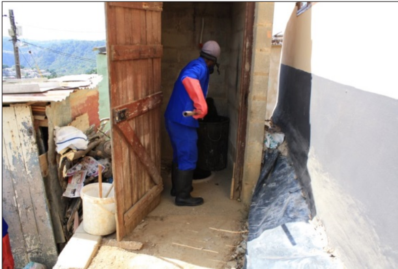
Manual pit emptying in eThekweni.
