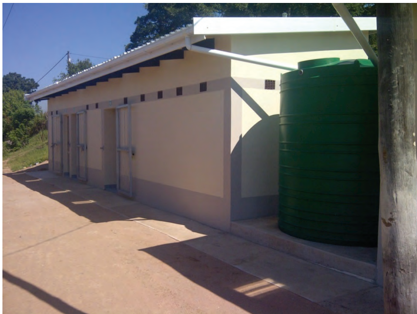
Figure 4.1 Newly built toilet blocks at Sizimesele Primary School
