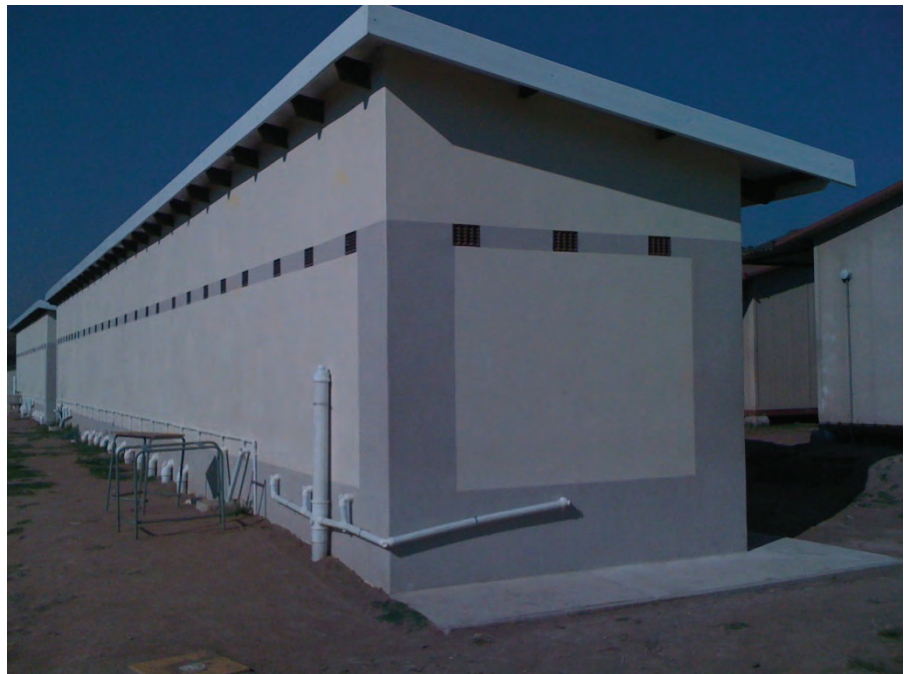
Figure 4.3 Toilet blocks at Thandaza High School
