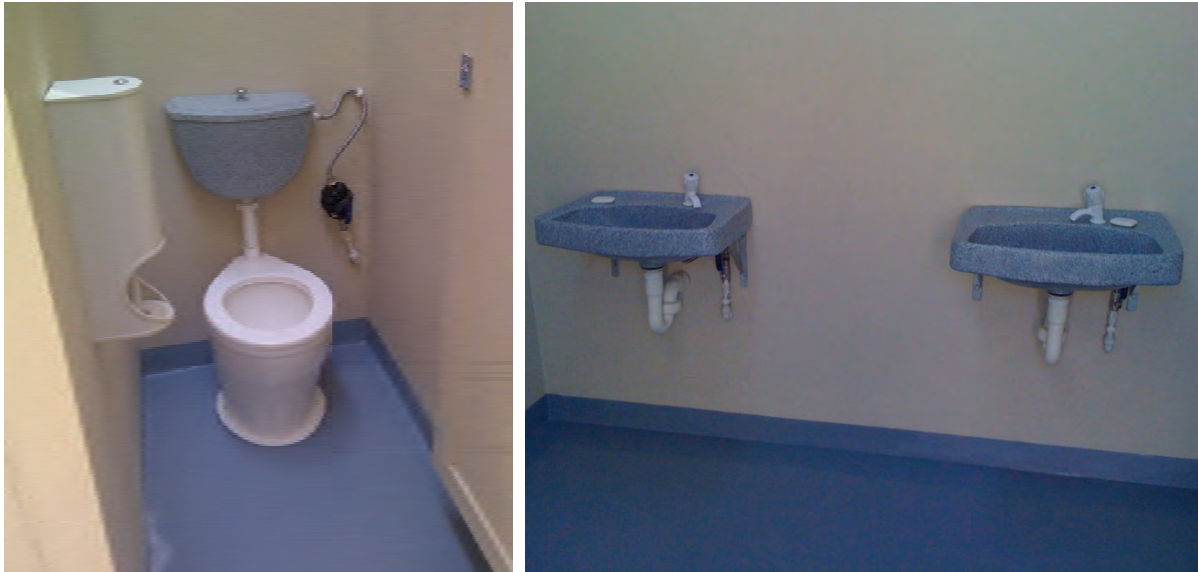
Figure 4.4 Stalls in the girls' toilets (left) and sinks in the women's staff toilet (right)
