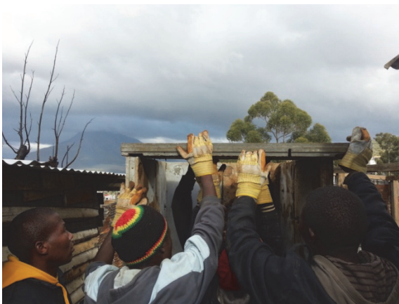
Figure 3.16: Placing the roof slab
