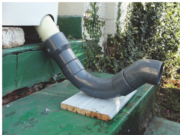
Figure 1.2: P-Trap Design (from Still & Louton, 2012)
