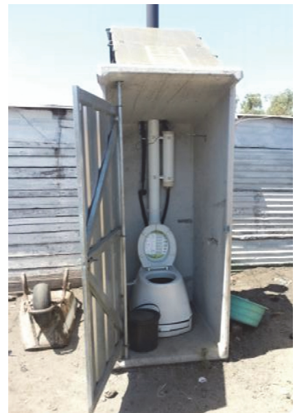
Figure 2.2: Existing EcoSan Toilets
