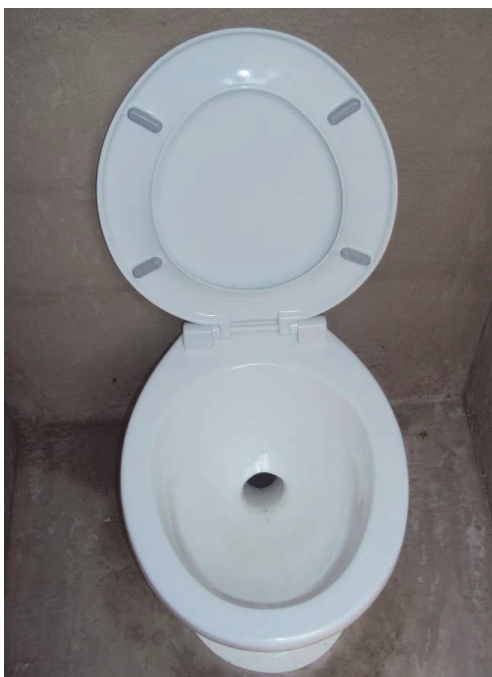
Figure 1.1: Pour Flush Pedestal (from Still & Louton, 2012)
