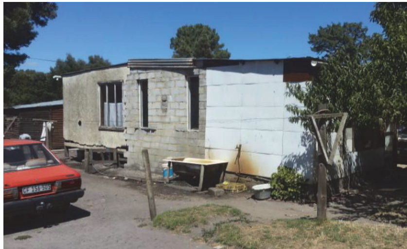
Figure 2.7: Typical View of Klein Begin Timber Building
