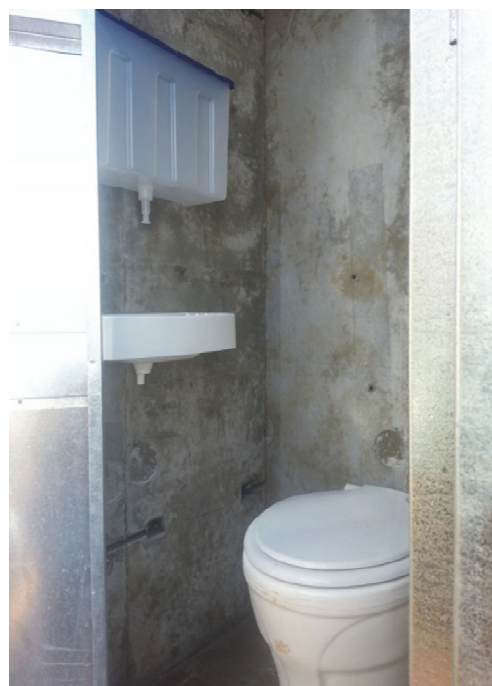
Figure 3.18: Toilet 1 complete with basin
