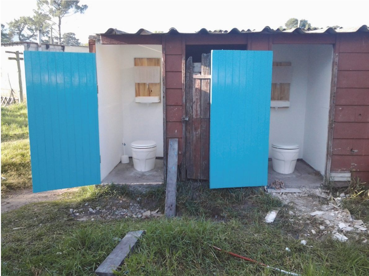
Figure 3.7: Toilets 3 and 4 complete
