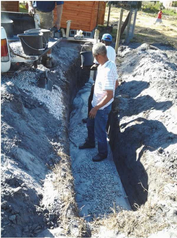
Figure 3.4: Constructing French Drain
