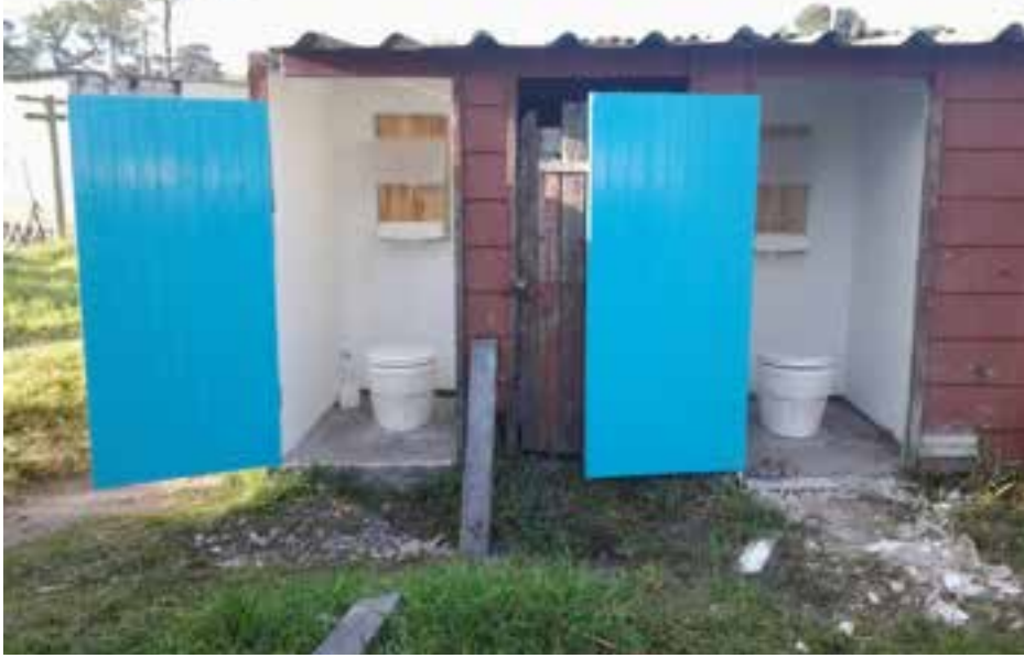
Toilets 3 and 4 complete
