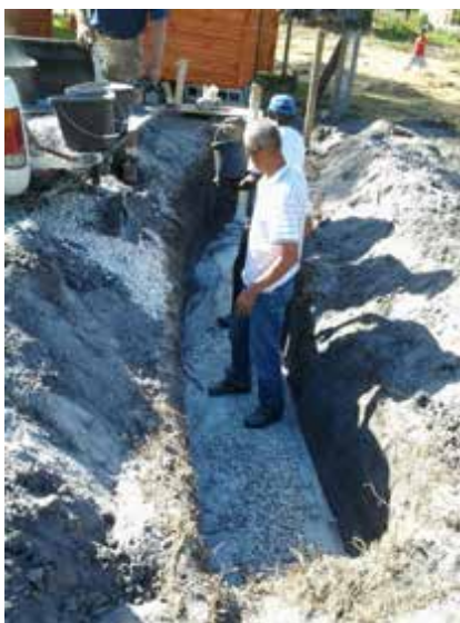
Constructing French Drain
