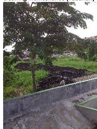
Figure 21 - Dried sludge after periodic cleaning maintenance (Tabanan)
