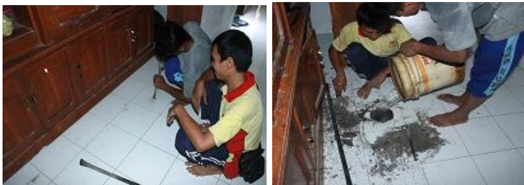
Figure 9 – Difficult access to pit under a house
