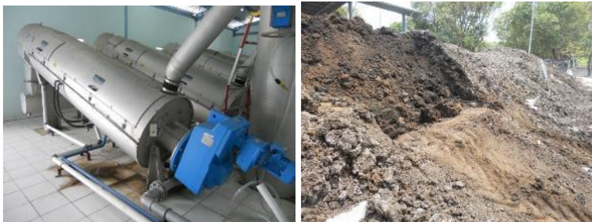
Figure 20 - Jakarta Huber screw press and Duri kosambi dried sludge from the screw press
