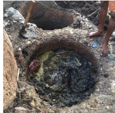
Figure 4: Manual faecal sludge collection (Credit: Arief Gunawan)
