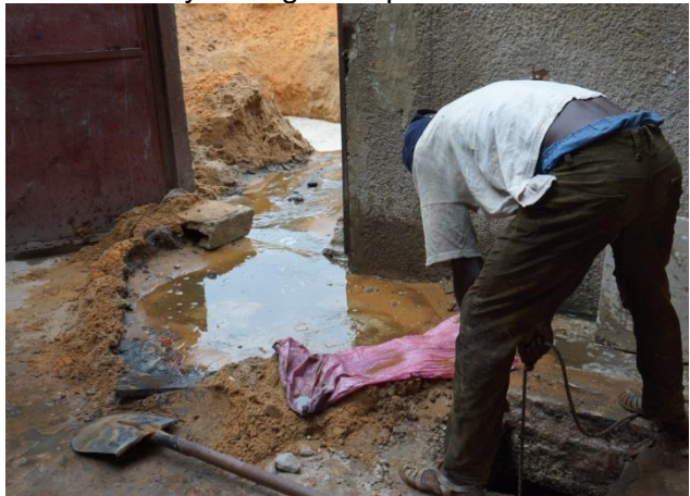
Figure 2: Manually faecal sludge collection and dumping in Dakar.
