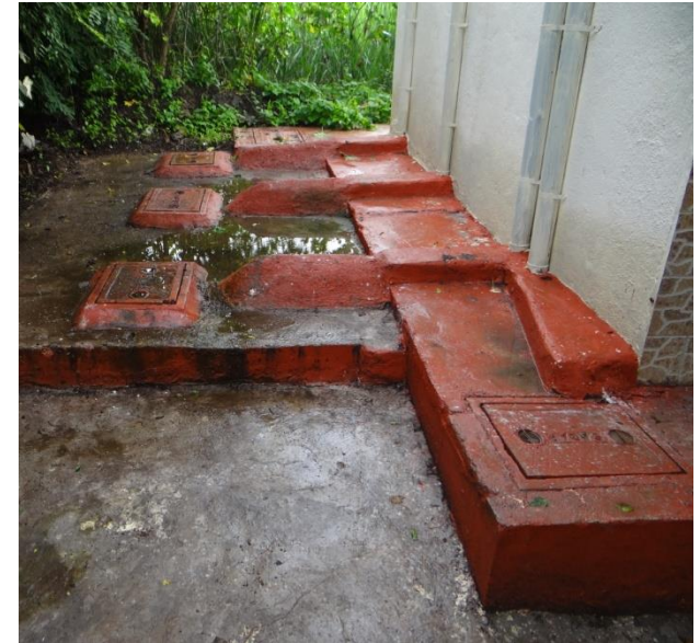
Sufficient size of septic tanks, with proper chambers and vents in new blocks
