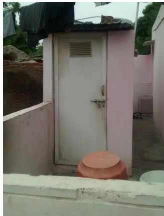
Private constructed toilet
