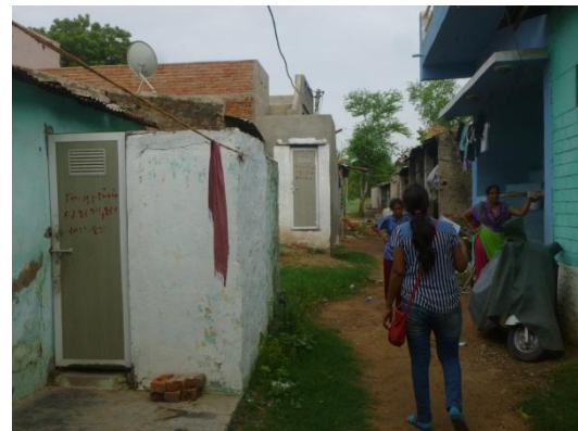
Inadequate space for twin pit
