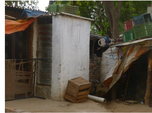
Toilet not connected with disposal system
