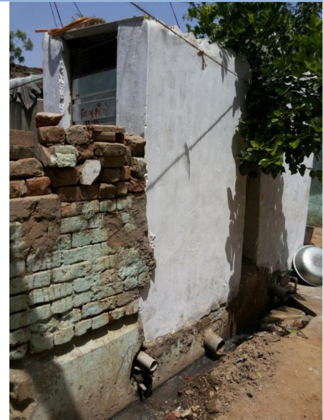
Individual toilets lack connection to disposal system
