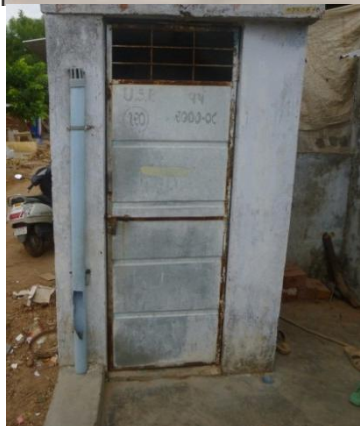
Single pit toilet
