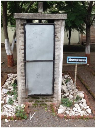
Brick, mortar with RCC roof and tin door
