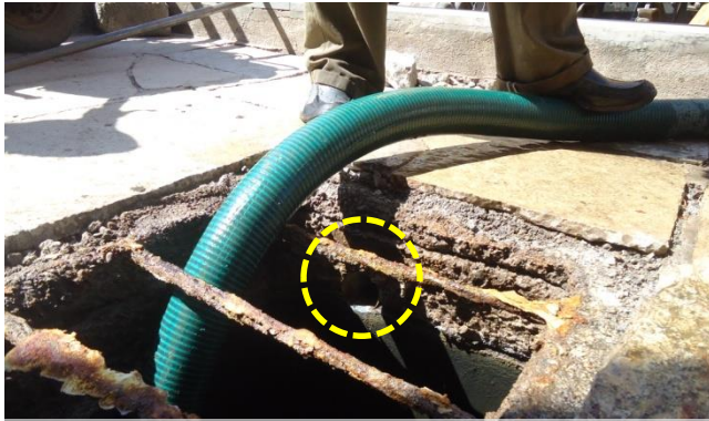
Case 4: Fulenagar, No proper design for inlet pipe
