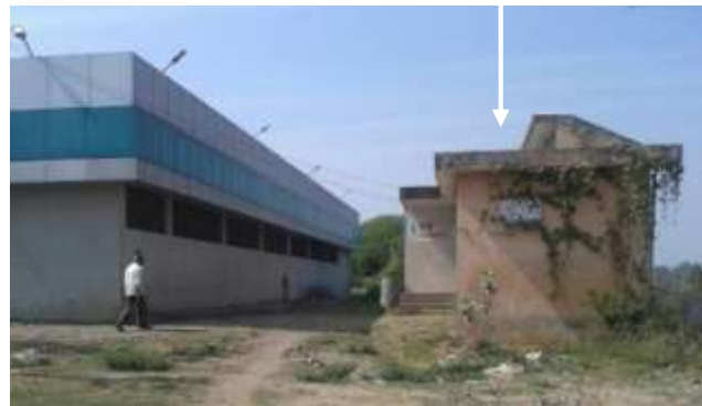
CT (12 seats) near DEWATS plant
