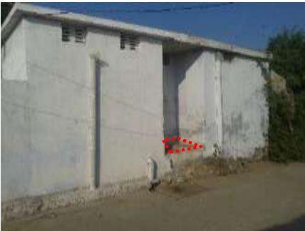
IHHL & Septic Tanks
