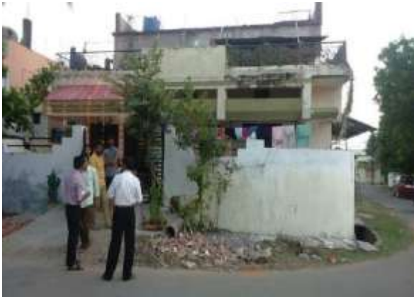
IHHL & Septic Tanks
