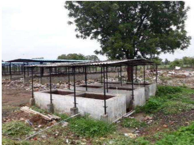
Vermi Composting Unit
