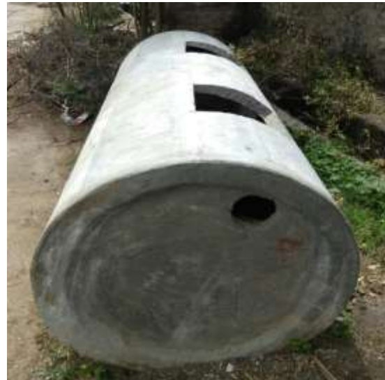
3 chamber with 2 opening precast septic tank
