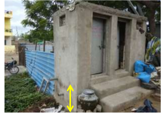
Inaccessible septic tanks with sealed tops
