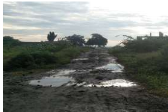
Spot along the internal road
