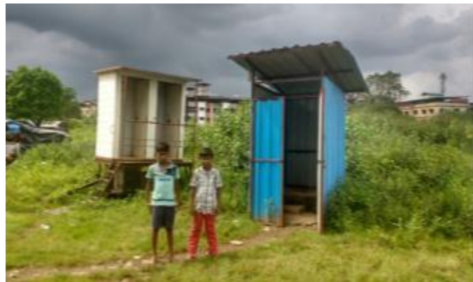
Mobile toilet at temporary settlement in Chiplun
