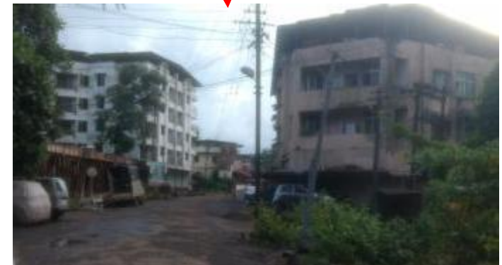
Large apartment buildings are a common sight.
