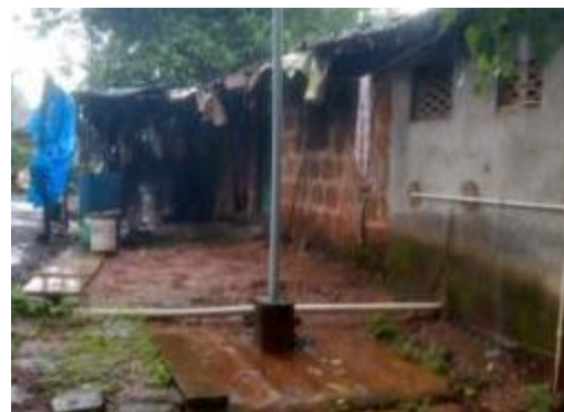
Unfinished semi-pucca structures are seen in a few areas
