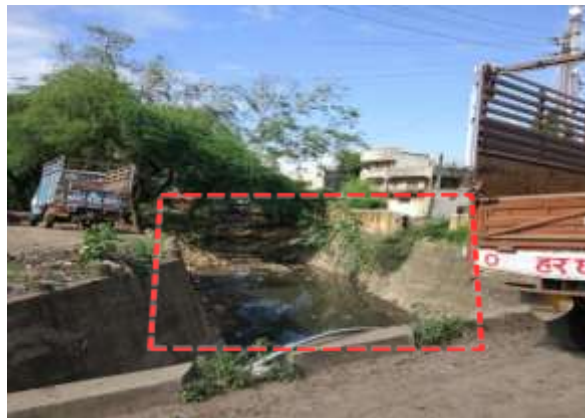
Nala carrying greywater to outside municipal boundary
