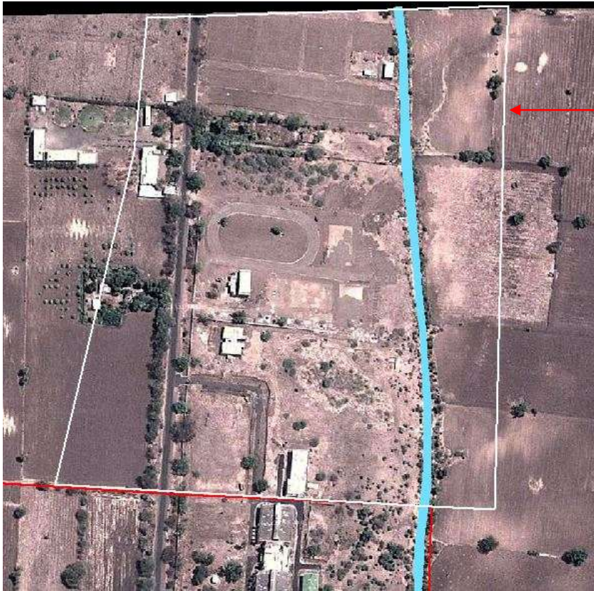
ITI college beyond the municipal limit towards the north along road to Melghat
