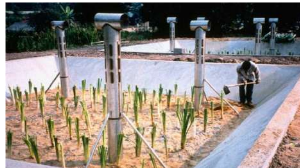
Planted sludge drying bed
