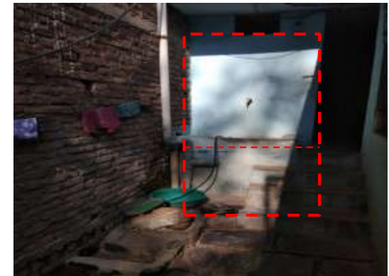
Septic tank in non-slum area
