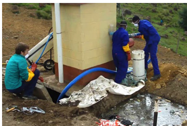
Emptying of pit latrine with vacuum pump. Photo by Mr Dave Still.
