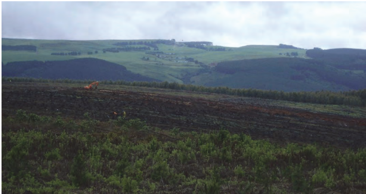
Figure 3.24 Commencement of sludge entrenchment at the Sappi site, November 2009
