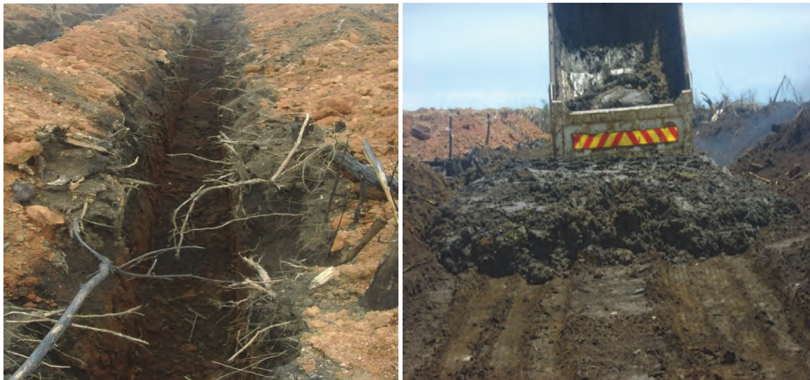
Figure 3.26 Prepared trench (left) and delivery of sludge from WWTW (right)
