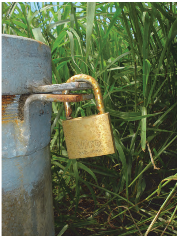
Figure 3 The tops of the wells were fitted with a lockable steel cap.
