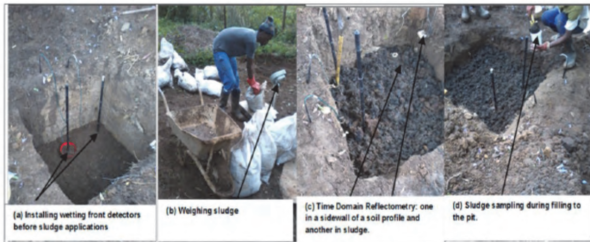
Figure 3.47 Installations of WFD and TDR and the subsequent weighing and filling of the sludge into the pit.
