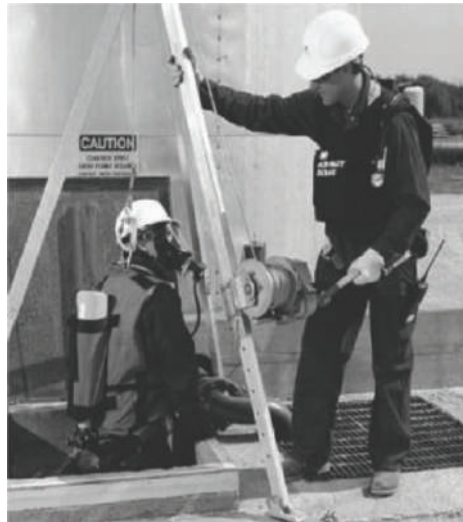
Figure 9.8 Photo showing typical confined space entry
