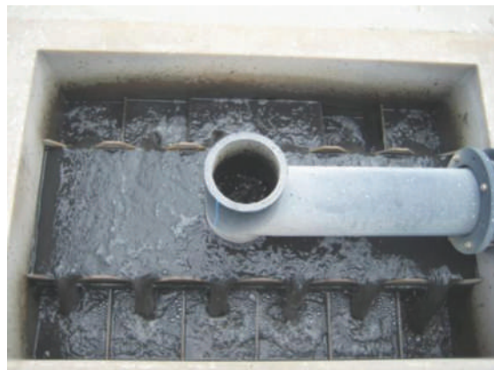
Cleaning of feed pipes by submersible pumps Clean feed pipes (equal flow distribution)
