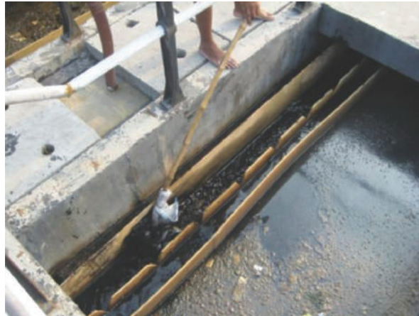
Figure 4.22 Cleaning of effluent gutters
