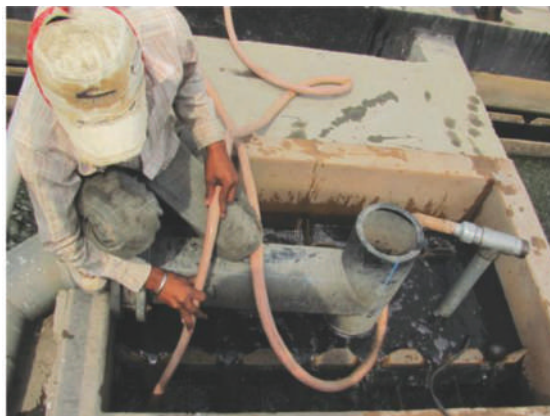
Cleaning of feed pipes by submersible pumps Clean feed pipes (equal flow distribution)
