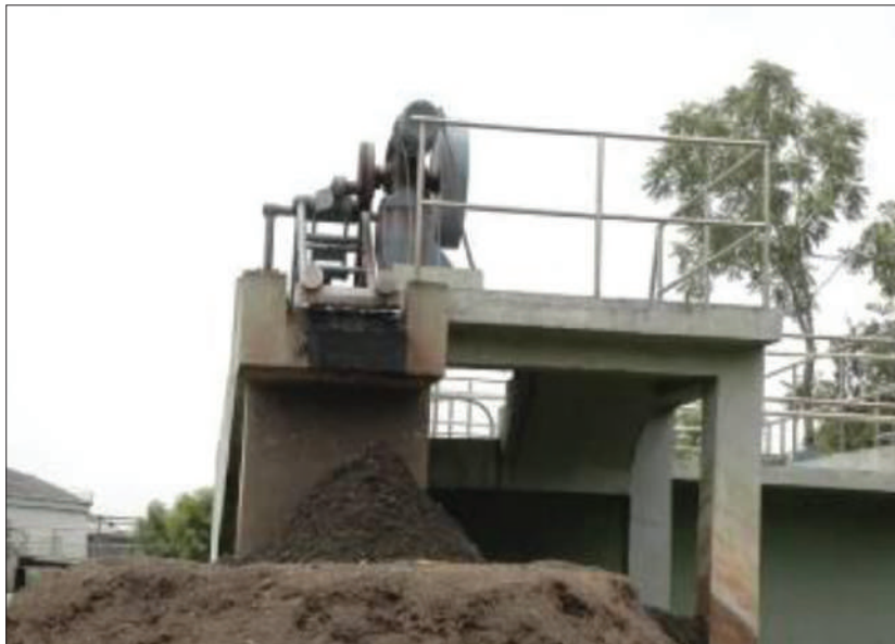
Figure 3.13 Typical grit chamber
