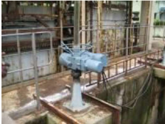
Figure 3.7 Electric motor driven gear actuator
