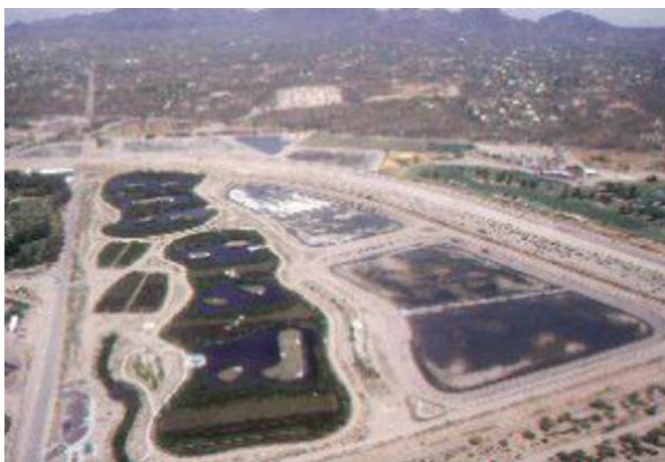
Figure A7.3- 15 Sweetwater SAT treatment plant, Tucson, AZ
