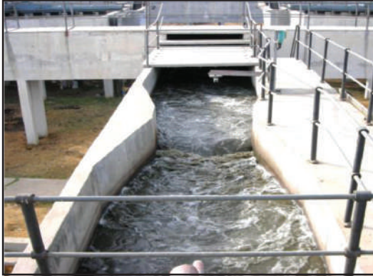
Figure 5.34 Typical Parshall Flume Installation
