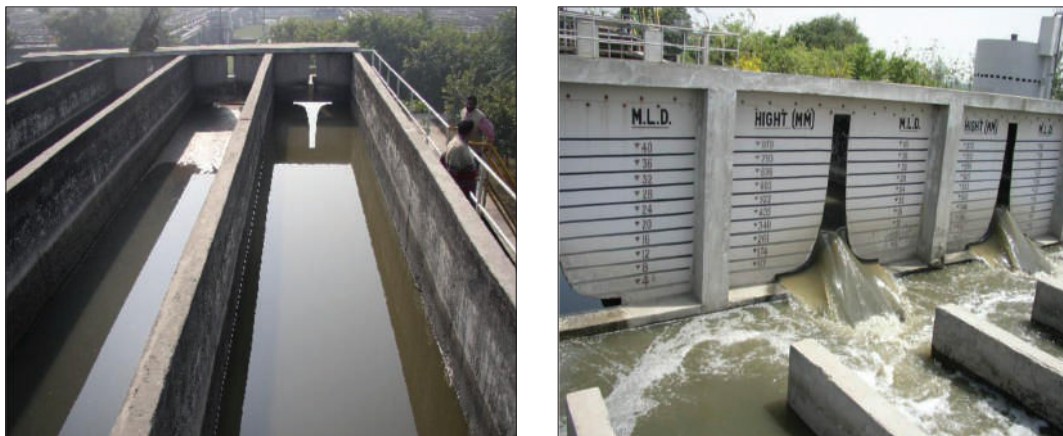
Figure 5.31 Typical Installation of proportional flow weir.
