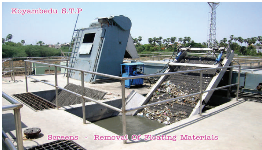
Figure 5.21 Mechanical screen with screen housing and ventilation at Koyambedu STP in Chennai. Manual screen and bypass channel screen in between the mechanical and manual screens is also seen
