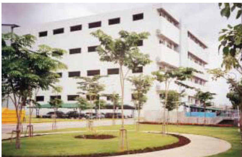
Figure 5.81 Yannawa STP, Thailand
