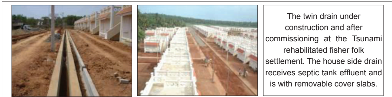
Figure 3.11 Twin drain system
