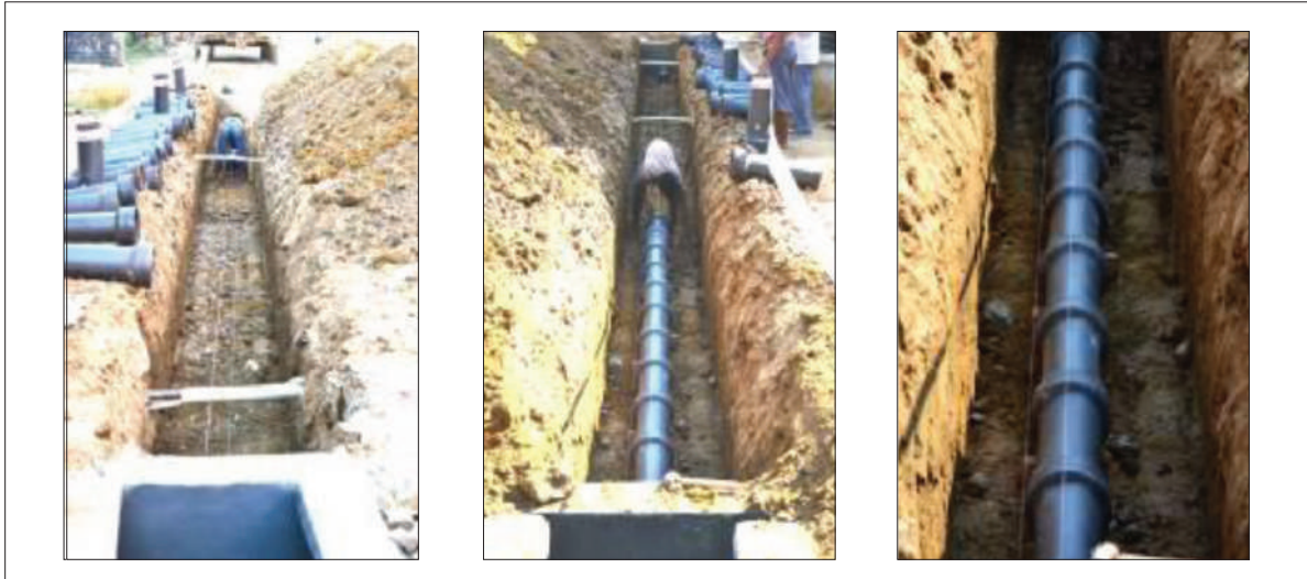
Figure 3.51 A simpler approach to initial laying and aligning the SW sewers by the two tight twines one on crown and one on mid diameter are used
