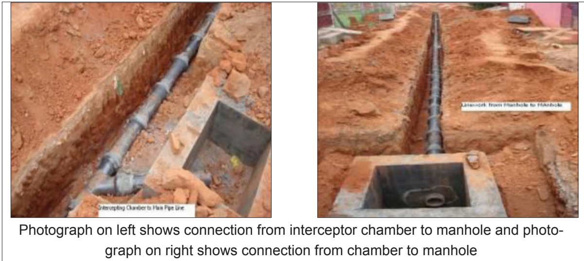
Figure 3.18 House sewer connections
