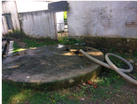
Figure 12: Desludging from a soak pit
