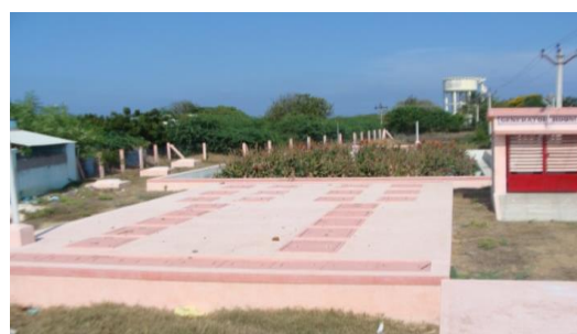
Figure 35: Anaerobic filter at Tsunami rehabilitation housing colony, India
