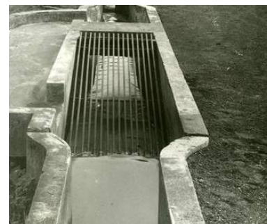
Figure 20: Screening Chamber
