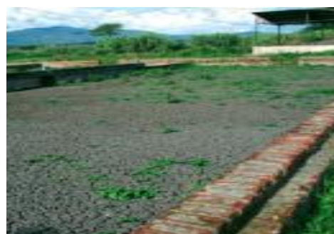
Figure 31: Sludge Drying Beds
