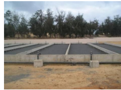
Figure 23 Sludge drying bed
