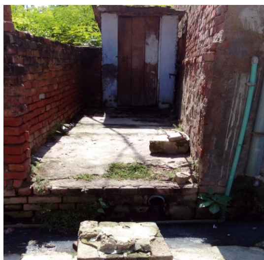
Figure 8: Toilet with Containment Unit
