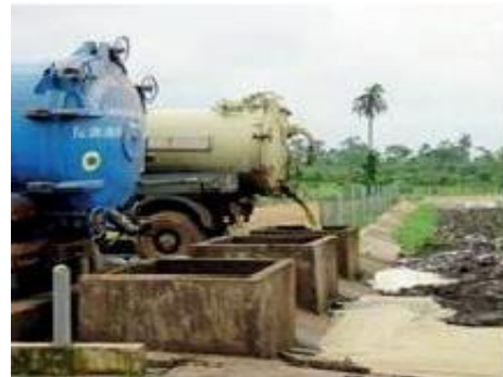
Figure 33: Septic Tanks in Ghana
