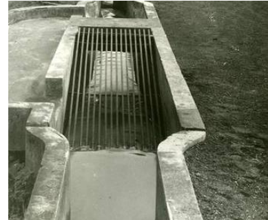
Figure 28: Screen and Grit Chamber
