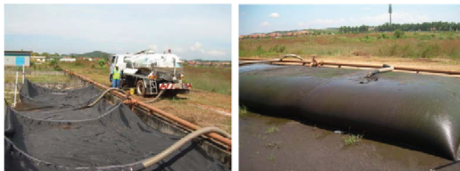
Figure 46: Geo-tube before and after use in Malaysia
