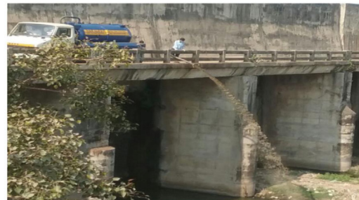
Disposal of septage in water bodies
