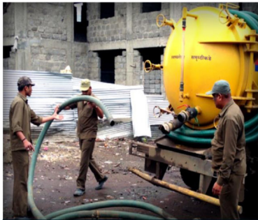
Unsafe handling of septage
