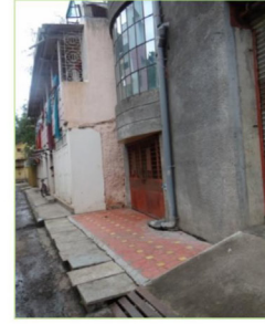
Septic tanks located near drains and sealed from the top
