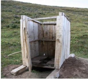
Single pit toilets
