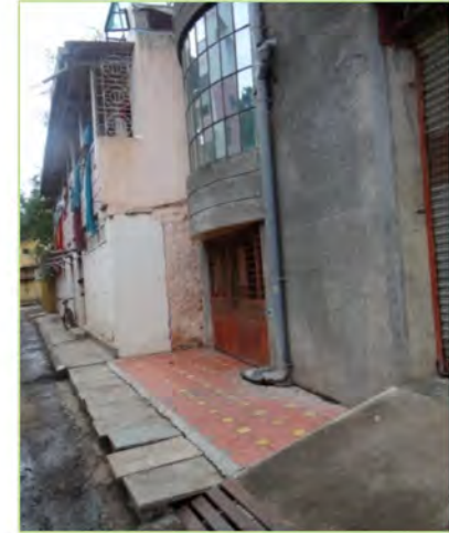
Septic tanks located near drains and sealed from the top
