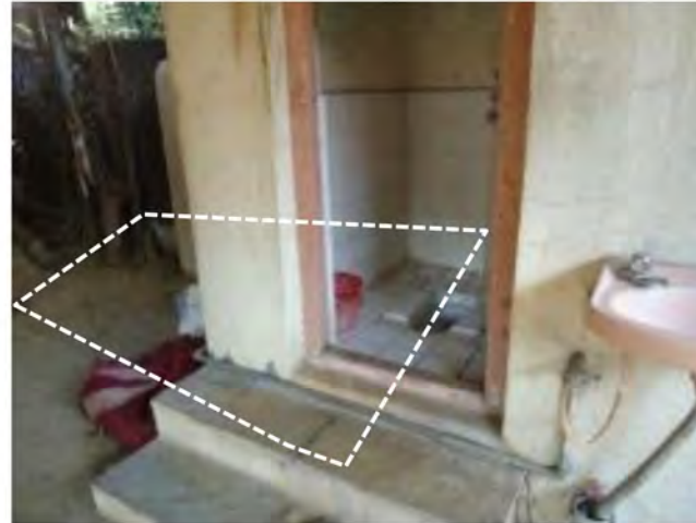
Inaccessible septic tanks with sealed tops
