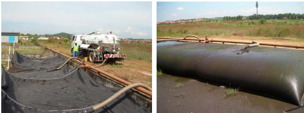
Figure 46: Geo-tube before and after use in Malaysia
