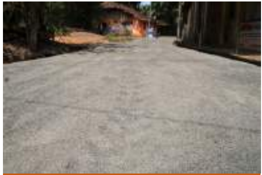
Road constructed from recycled plastic
