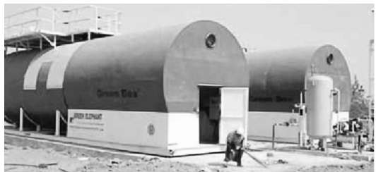
Electricity generation plant
