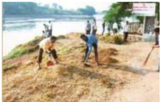
Council undertaking the cleaning of river bed
