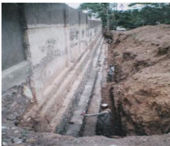
Repair work in progress
