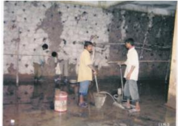
Repairing and cleaning of the Water Tank 1
