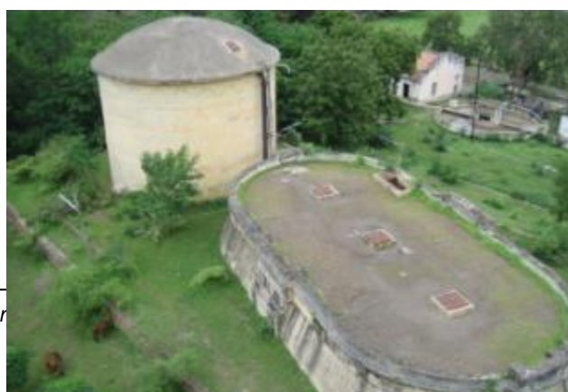
Storage Tank at the Filter Plant
