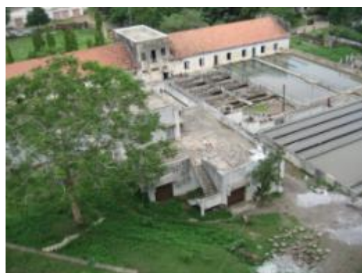
Takhteshwar filter plant
