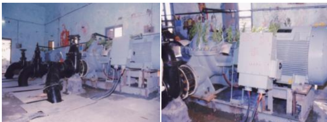
Sarkadia Pumping Station
