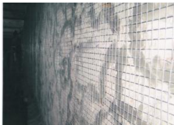
Wire meshing as Reinforcement
